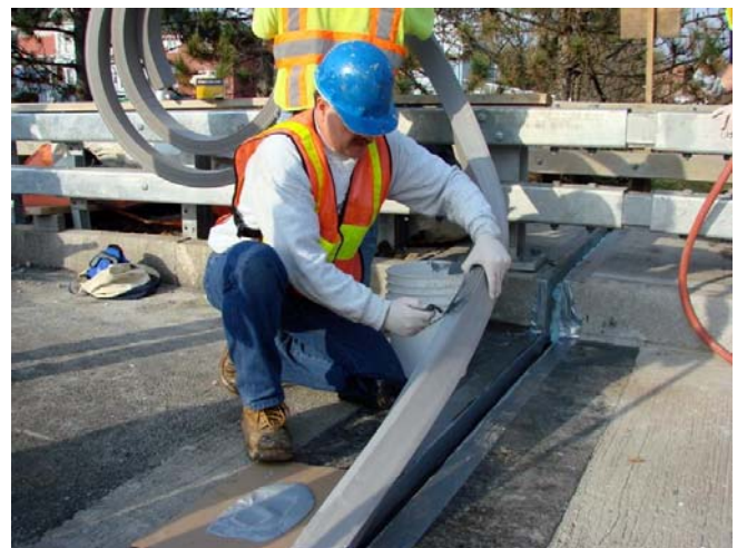
Installation of IAS Series using Pro-Bonder and unique installation tools. Remove epoxy adhesive from top of seal prior to cure to allow the seal to move freely.
